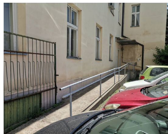
Photo 4: accessible entrance in the basic court in Pirot
